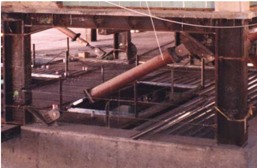
Figure 7: Diagonal Brace FVD Configuration
