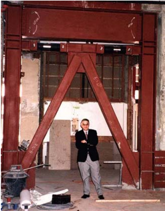
Figure 9: Horizontal FVDs on Chevrons
