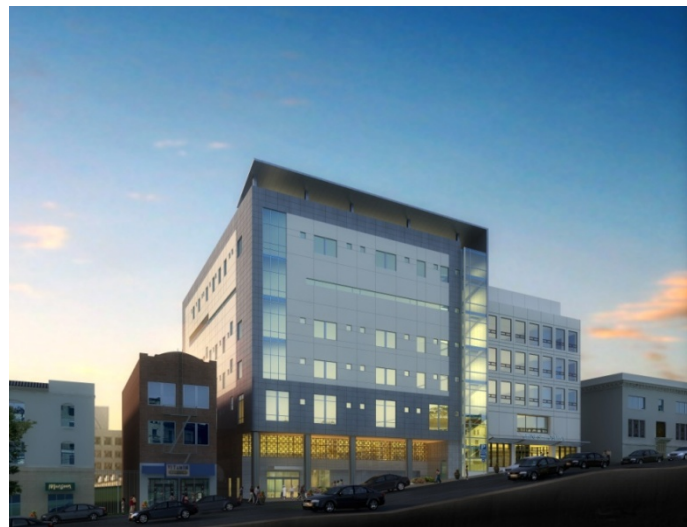
Figure 2: Exterior view of New Acute Care Hospital and surrounding buildings
